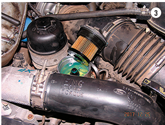
SECONDARY FUEL FILTER with the top removed. The top was removed to see if the electric fuel pump would pump fuel.
