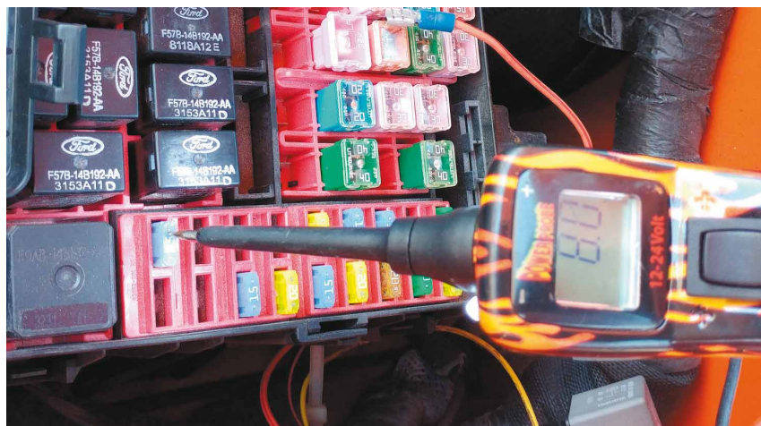
VOLTAGE DROP STILL evident through the fuse after yellow wire has been removed from the fuse socket.
