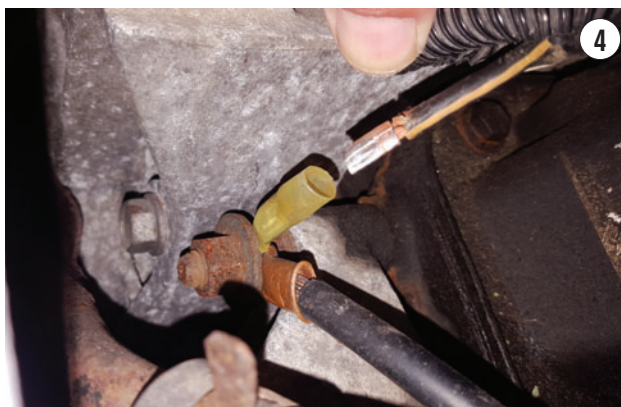
TOUCHING THE GROUND WIRE caused the substandard repair to fall apart.
