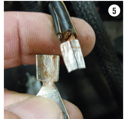
THIS CONNECTER was not even crimped or soldered together.
