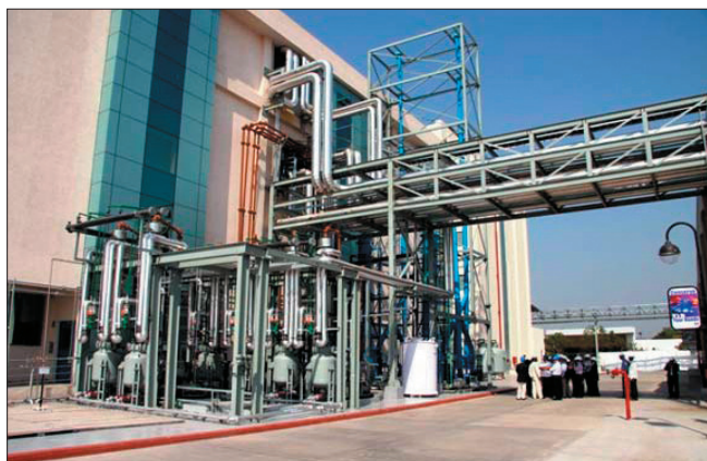
Dishman manufacturing plant
