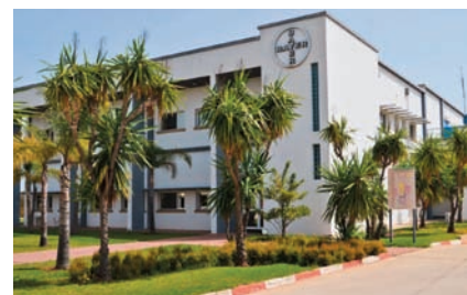
Bayer's manufacturing plant
