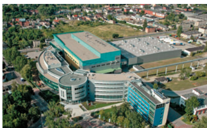
Polpharma manufacturing plant
