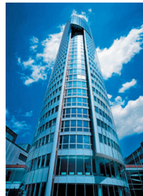
Floridotower, Pfizer offices
