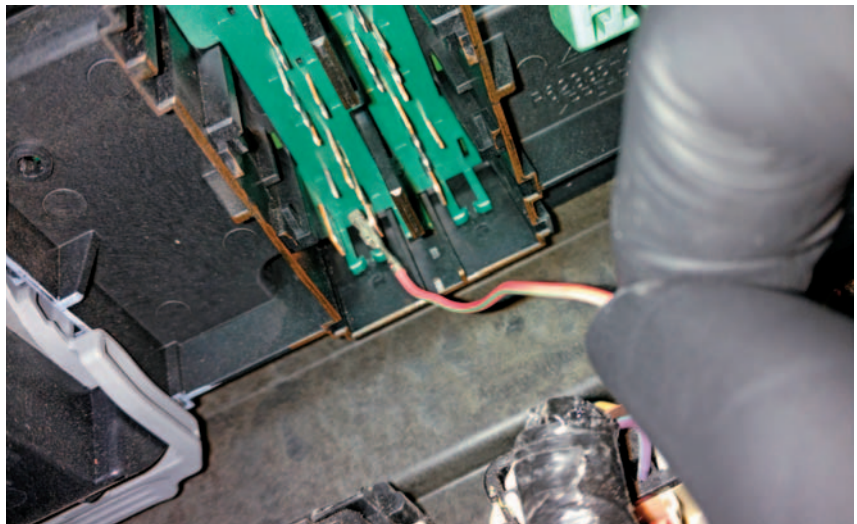
THIS IS HOW LOOSELY THE TERMINAL fit onto the mating male pin at the TIPM. A correctly fitting terminal will not wiggle and exhibit a drag when sliding on the mating pin.
