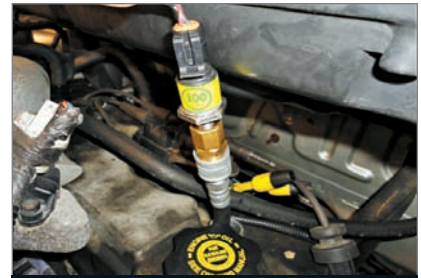
Pressure transducer being used for diagnostic purposes.
