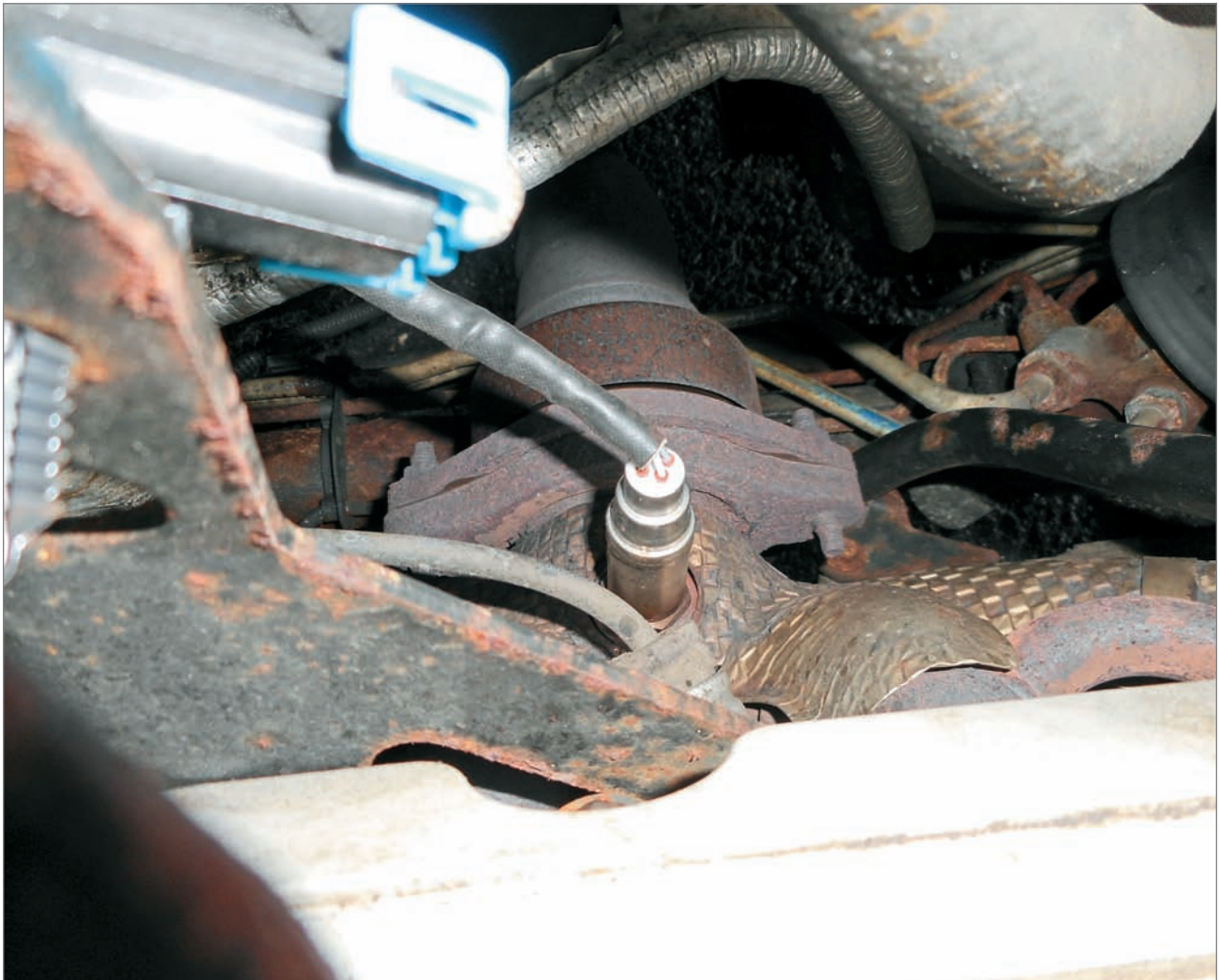
Both of the oxygen sensor grounds had excessive voltage drop and were ignored by the ECM, which suspended the monitors using the sensors for test purposes.
