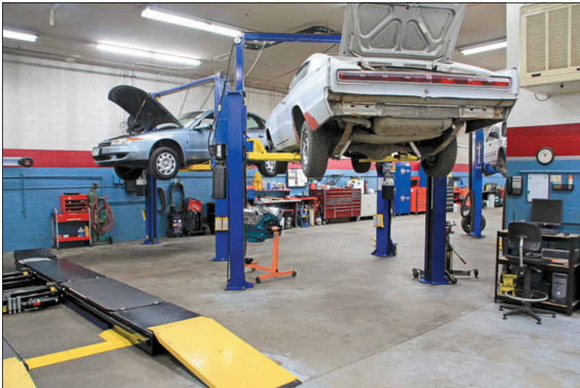
Here is a view of the south side of the service bay, featuring an alignment rack and three bays with two lifts.
