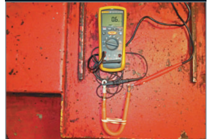
Here I wanted to simulate a bad (shorted) cable reading. Replace cables that have failed; never try to repair one.
