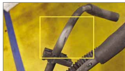
Simple problem. Aged secondary wires intermittently allowing high voltage to leak to ground. Visual inspections come first!
