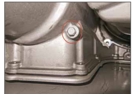
This is a GM check plug. Seems easy enough, but if the fluid temperature isn't right you may actually let fluid out that needs to stay inside.
