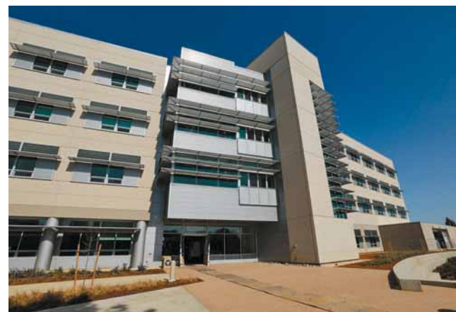
>>> The 76,000-square-foot, four-story Veterinary Medicine Research Facility 3B at the University of California-Davis will be dedicated to making discoveries in basic science as well as human, animal and environmental health.
