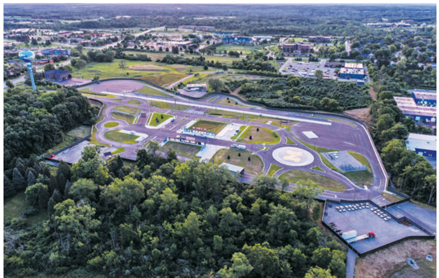
AN AERIAL VIEW OF THE MCITY TEST FACILITY , which sits on a 32-acre site and features about 16 acres of roads and traffic infrastructure.
