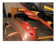
HEAT CURE THE REPAIR AREA TO ELIMINATE READ THROUGH.
