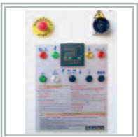
Electromechanical control panel.
