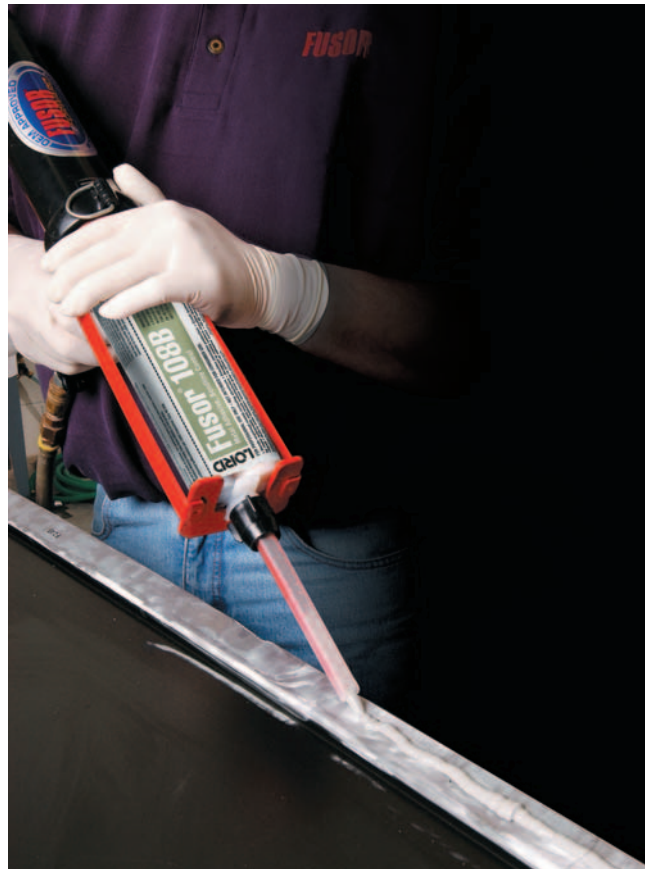
FUSOR 108B is an example where Ford chose to use a non-crash durable adhesive in conjunction with rivets for structural repair.
