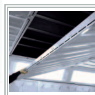
Hinged ceiling filter frames for easy replacement of 10 micron media filters.
