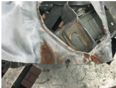
RIGHT APRON BAFFLE with excessive corrosion and body filler
