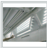
Eight 6-Tube light fixtures with hinged access for ease of cleaning and maintenance.
