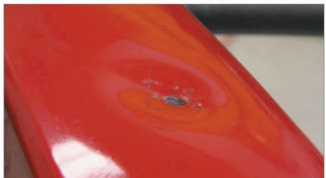
Structural damage to unreinforced substrate.
