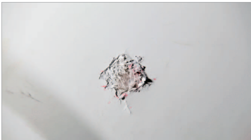
Damaged fibers in reinforced plastic before repair.
