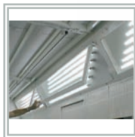
Eight 6-Tube light fixtures with hinged access for ease of cleaning and maintenance.
