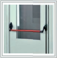
Internal push bar on the front door and the side personnel door.
