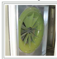
Pre- and Post-filtration: Intake and Exhaust. Two direct drive centrifugal fans with 2 sets of 10 bag filtration for each.
