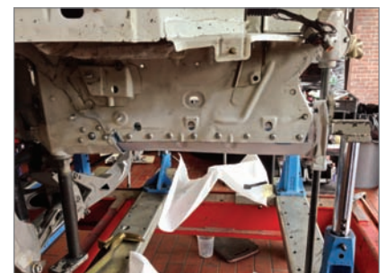
Flow Drill Screws (FDS) installation with structural adhesive (blue glues) on outer rear lower uni-rail
