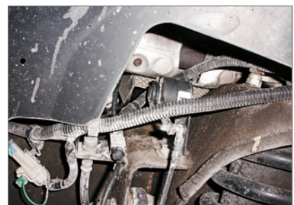
One of the most common failures in electronic ride control is the body/suspension sensor. This Cadillac Escalade uses a snap-on sensor link that can be dislodged by large ice chunks when driving in winter.
