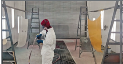
Testing compressed air versus nitrogen using a low-hiding yellow color. The nitrogen proved to help the color cover more quickly.
