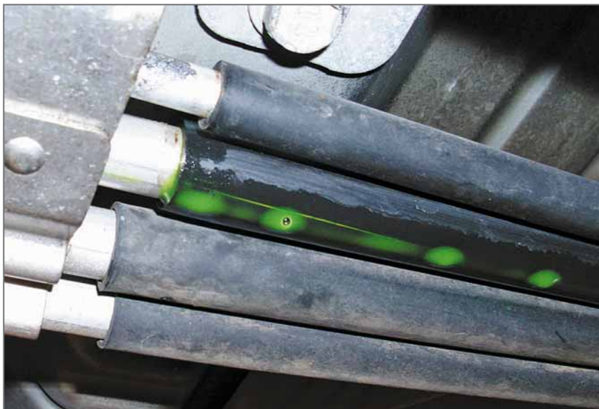
Be wary of pinholes hiding under line wrappings.
